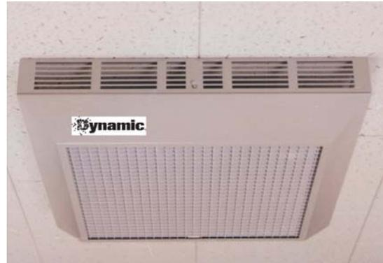
The Dynamic OH1010 Overhead Air Purification System will remove the smallest sub-micron particles (97% at .3 microns) in addition to odors and gasses and offers an excellent solution in applications where tobacco smoke is present. Polluted air is drawn in through the bottom return grille and purified air is expelled through the cabinet side louvers.
